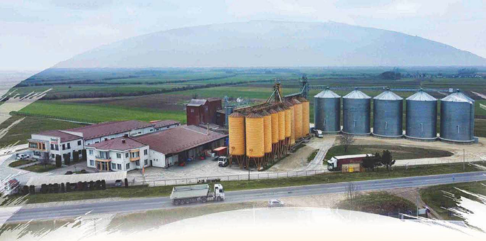
Manufacturing facility in Salas Nocajski
